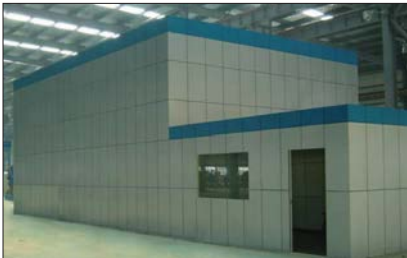
Shielded room for 110kV cables(High Volt equipments)
